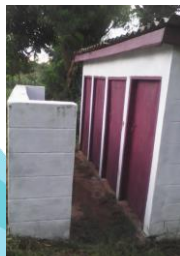
Latrine block built for BONGGS in 2017, using £2,500 raised by the Church
