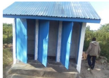
Latrine block built for the Primary School in 2021, using £2,000 raised by the Church
